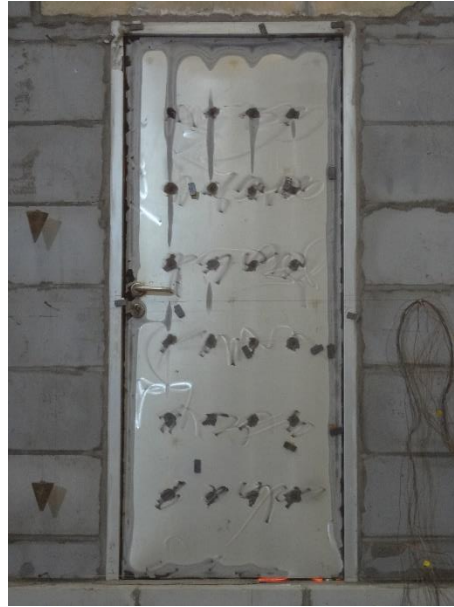
Fig. 9 Unexposed Side after 70 Minutes
