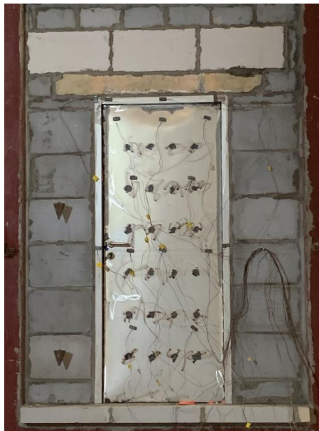
Fig. 6 Unexposed Side after 40 Minutes
