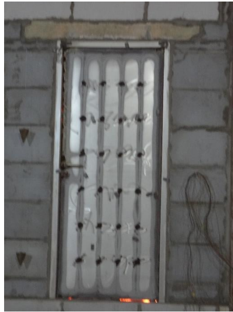
Fig. 21 Unexposed Side after 190 Minutes
